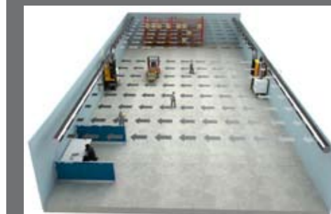
System Push-Pull z dwoma filtrami i dwoma wentylatorami
